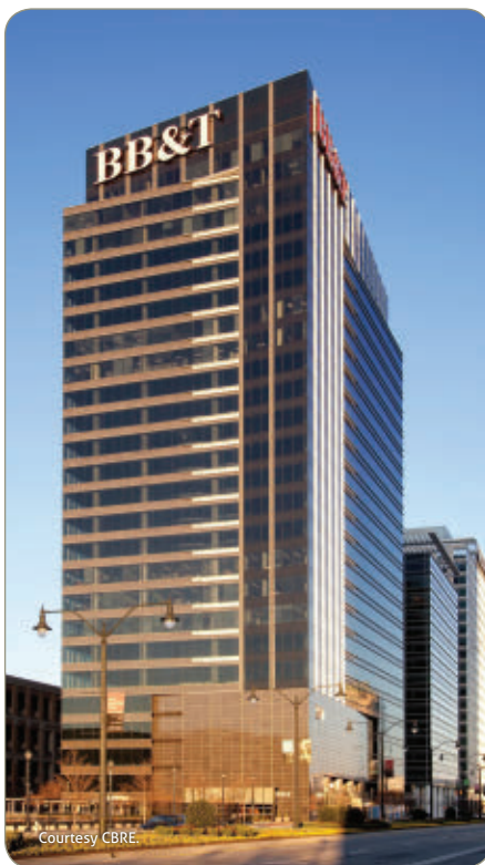
The 271 building was the first Atlantic Station high-rise to boost HVAC system performance with precision control valves.
